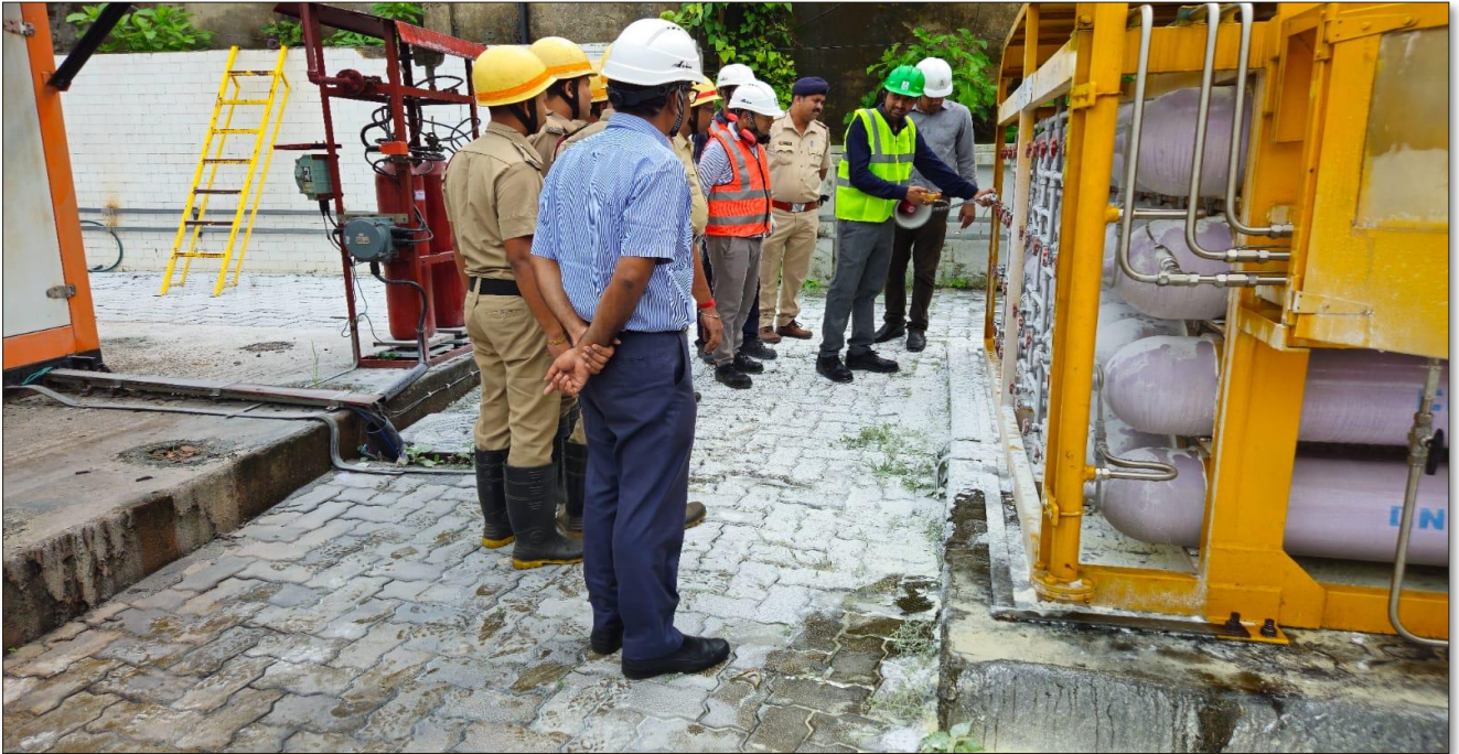
7. Gas Leakage Checking by Safety Officer in presence of SIC, Head (CA & CO and HSE), and District authorities
